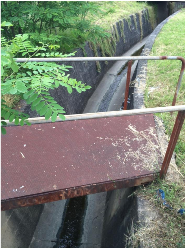
Plate 3-5 Channel at Downstream end of Site
